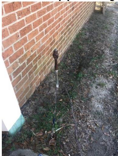
No, pipes like the one pictured are not connected to a heating oil tank. Many residents have asked about pipes that look like the one pictured here. These pipes are decommissioned and were used to meter natural gas. Natural gas was once used at Laurel Bay, but has been replaced by other heating sources.
